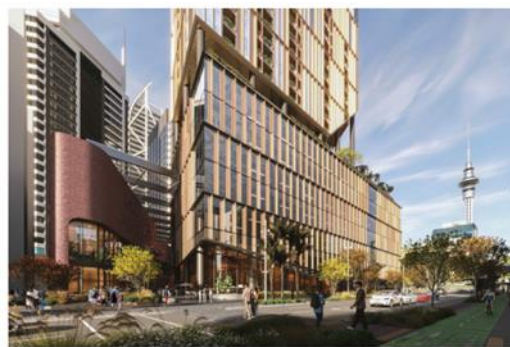
Figure 2.34 Podium (P3 at left, P2 at right) viewed from the north-west over Lower Hobson Street, shown with the existing ramp removed. (Render 09)
